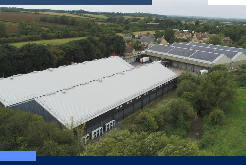
Ducklington Mill, a key hub for Phillip Dennis Foods in Witney, aimed to boost sustainability by installing a photovoltaic (PV) system. However, the cold storage and warehouse roofs were outdated and unsuitable for PV installation. Central Group was brought in to refurbish both roofs, making them PV-ready and enhancing the facility's functionality.
