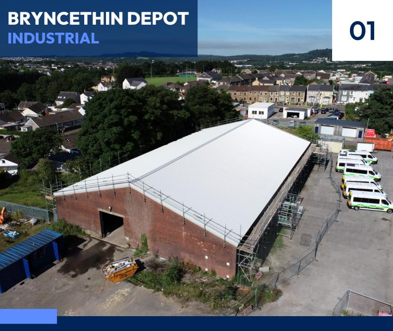
Central installed a new metal roof for Bridgend County Borough Council at Bryncethin Depot. This industrial building measures 1,144m² and is located in Bryncethin, Bridgend. The asbestos cement roof and rooflights had passed their serviceable lifespan, making the building unfit for use.
